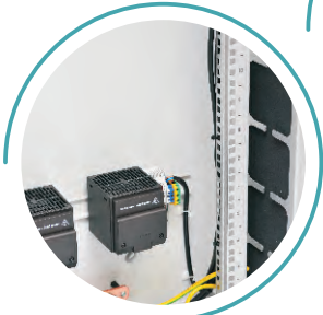
Heating of cabinet via heater with thermo ventilator.
