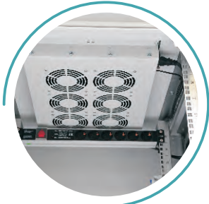
Cooling of cabinet via 6-ventilator ventilation panel.
